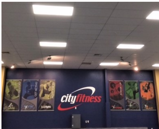
EDGE LIT PANELS AT CITY FITNESS NEW PLYMOUTH
